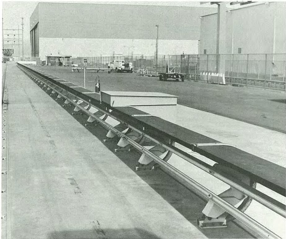
Figure 2-8. 500-Foot Test Track, Chula Vista, California
